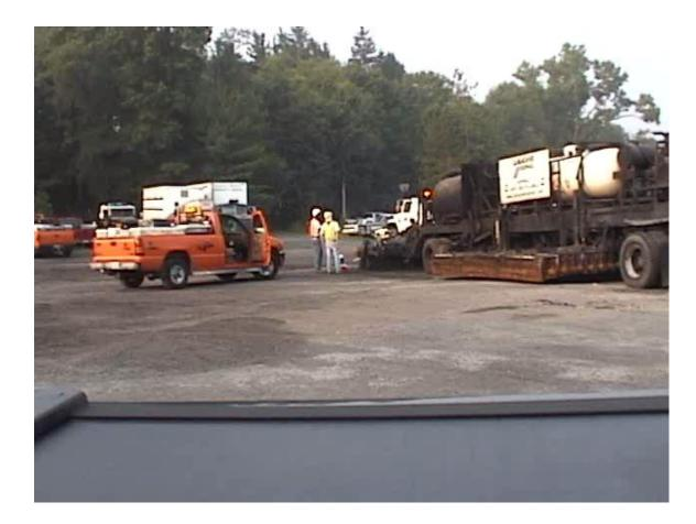
1<sup>st</sup> Pre-Heater takes pavement temp to 180 – 200 degrees
