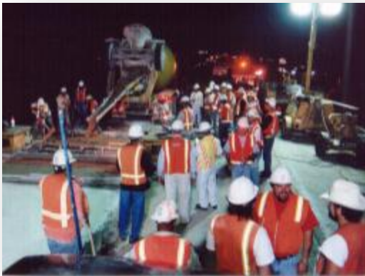
Pavement replacement at I-10, Pomona, CA, 1999 (4-hrs RSC)
