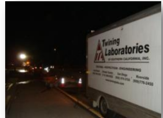
Pavement replacement at I-710, Los Angeles, CA, 2005 (1.5-hrs RSC)
