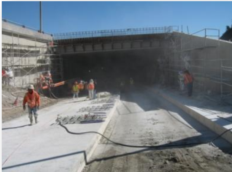
Emergency rehabilitation of truck bypass tunnel (after vehicle fire) I-5 and CA-14, November 2007.
