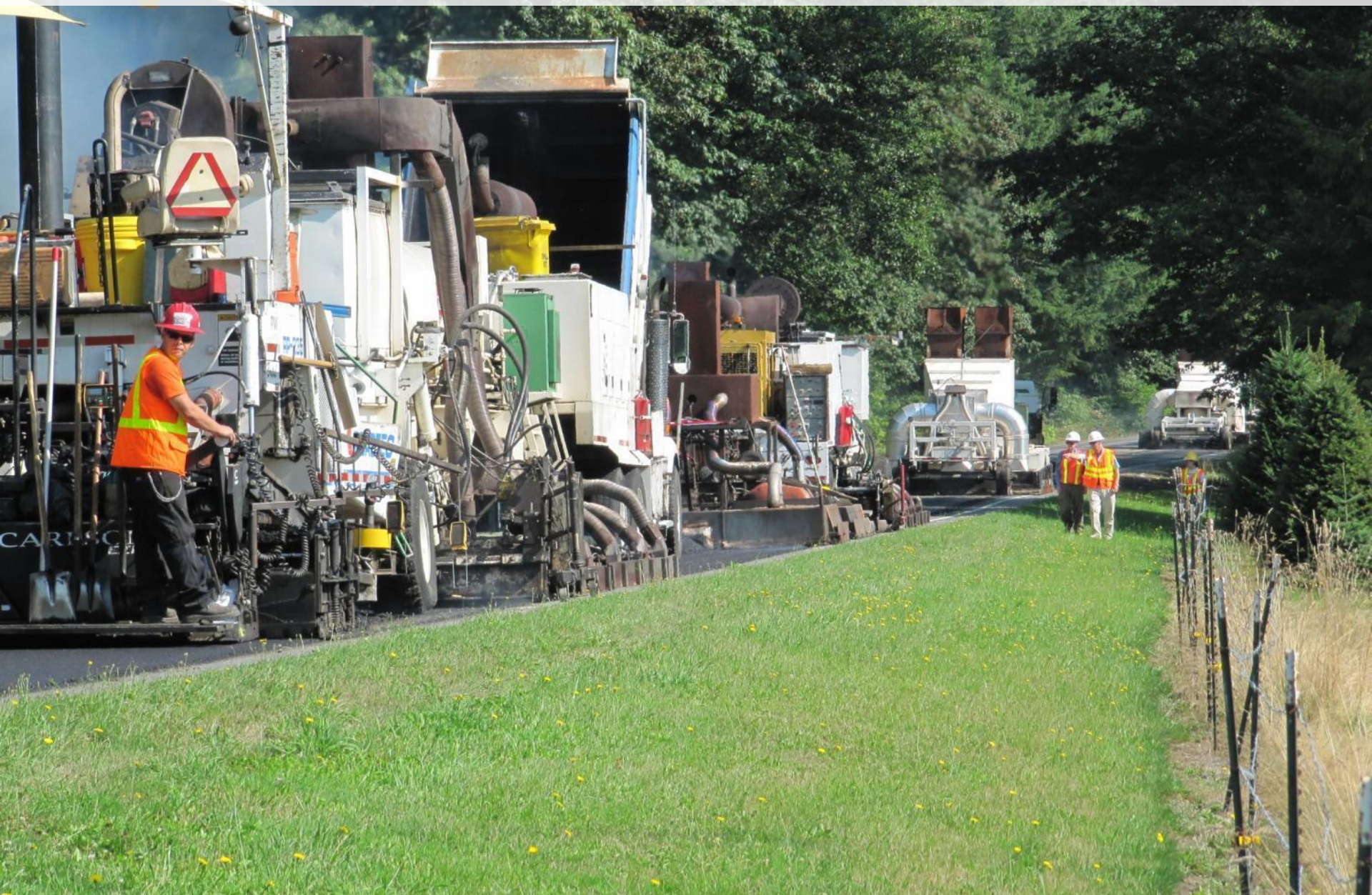
Hot in-place recycling on SR 542, Washington, United States
