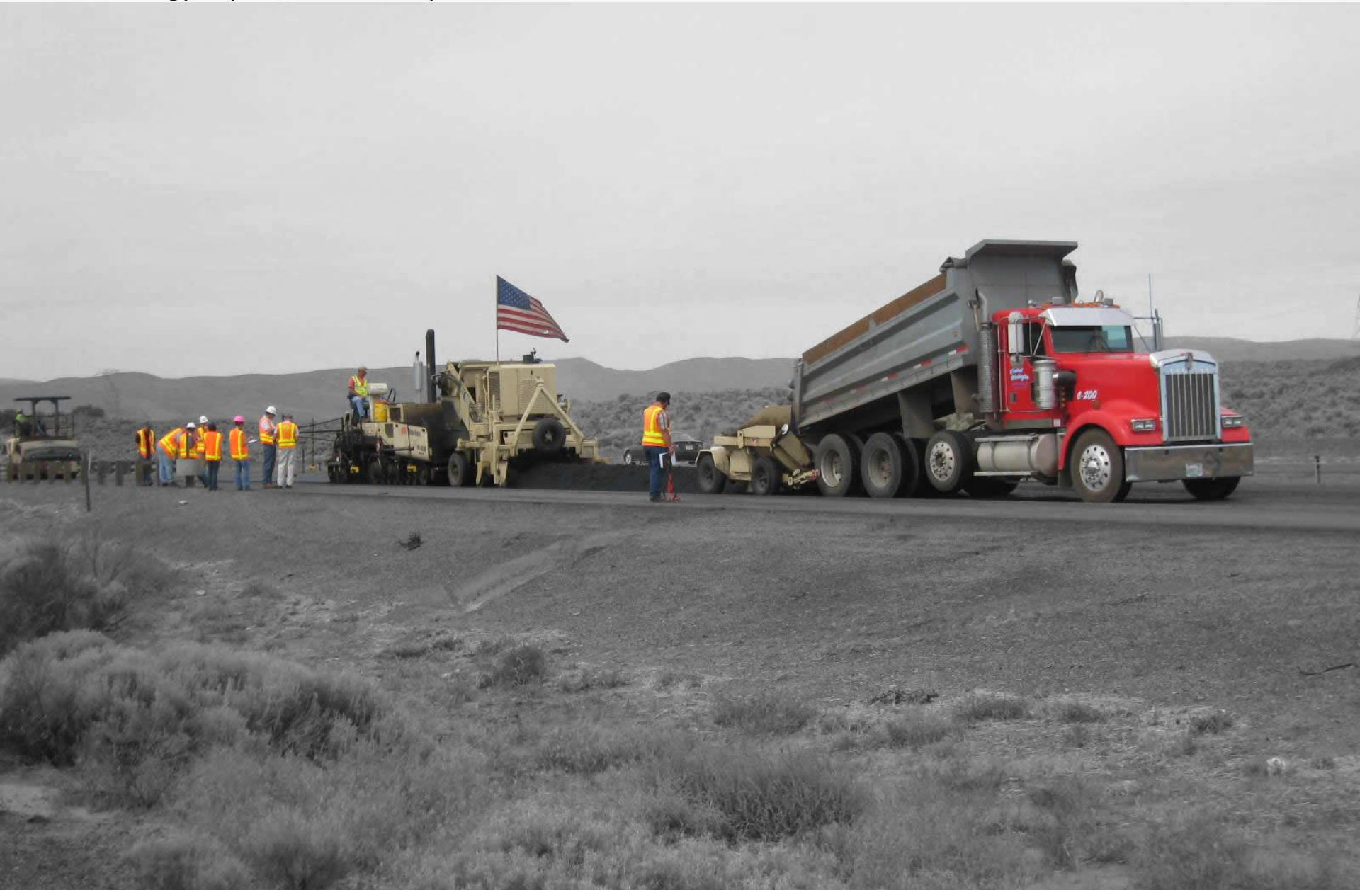
Paving Sasobit warm mix asphalt on I-90 near the Columbia River, Washington, United States
