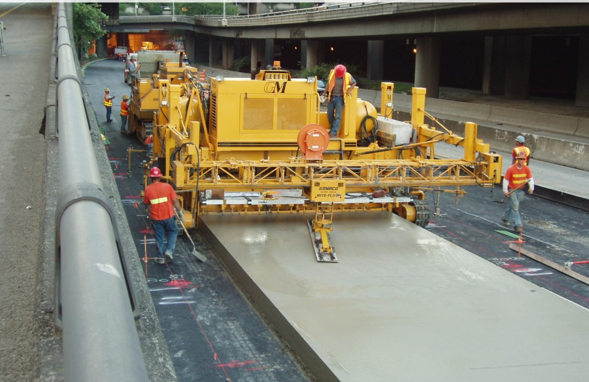
Paving 13 inches (330 mm) of jointed concrete pavement on I-5 in Seattle, Washington, United States
