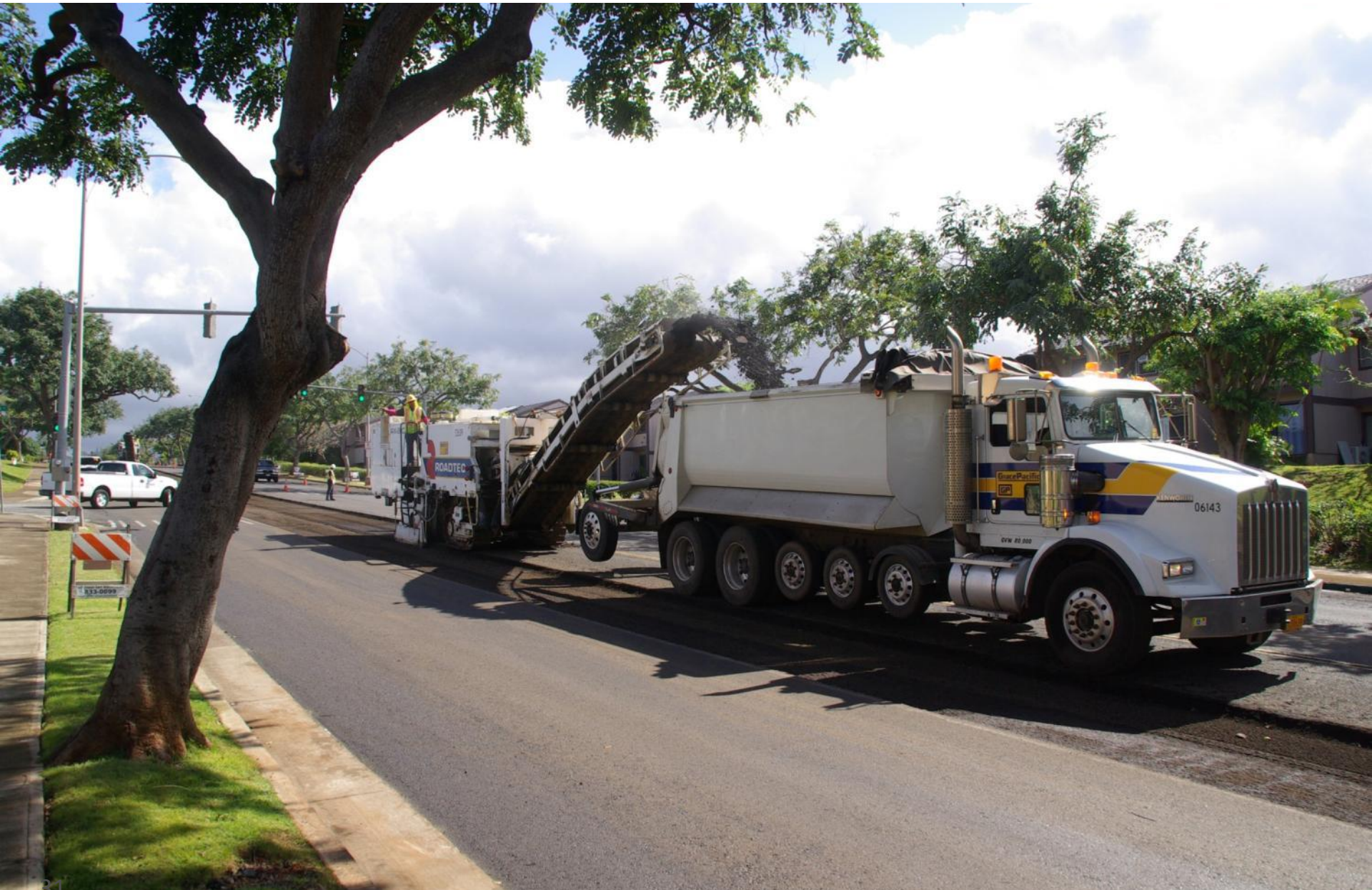
Milling up existing HMA surface, Ka'ahumanu Rd., Pearl City, Hawai'i, United States
