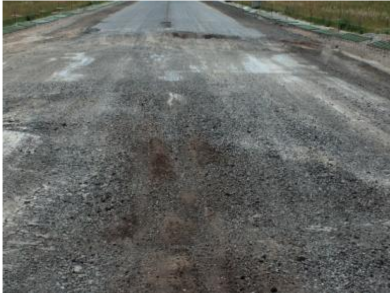
Removed 6 in of existing 9-in HMA Pavement
