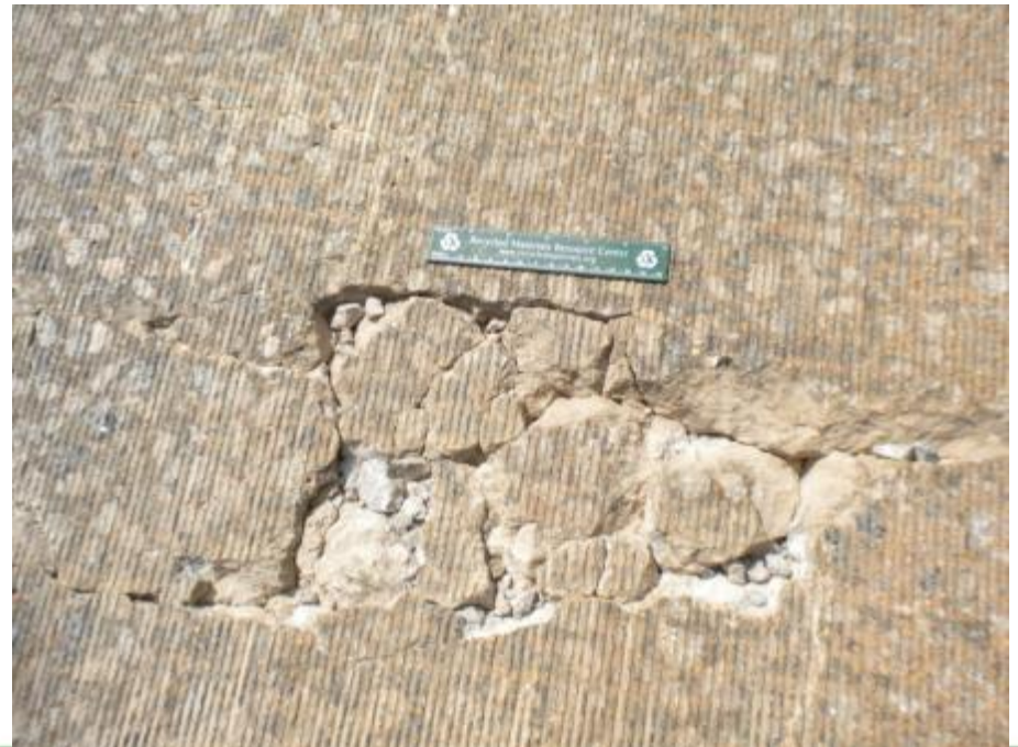
Failing Concrete in Quiet Concrete Section
