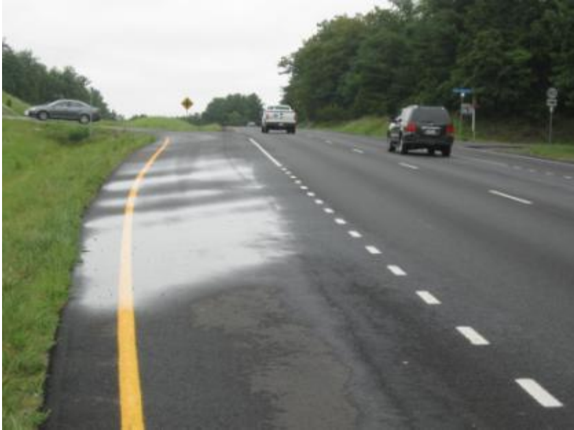
PFC's with Parallel Conventional Pavement
