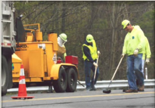
Crack Sealing
