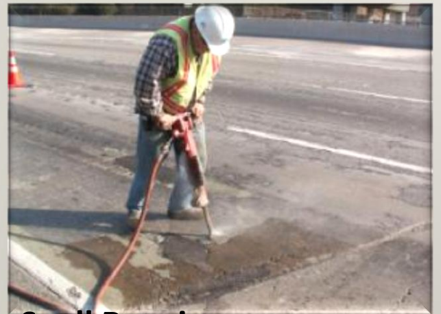
Spall Repair
