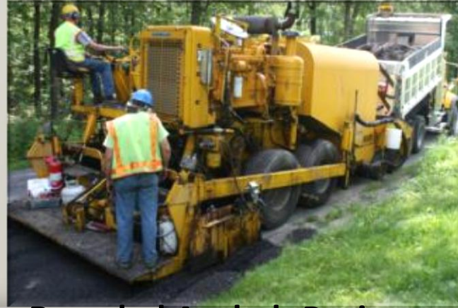
Recycled Asphalt Paving
