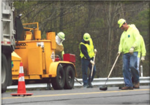
Crack Sealing
