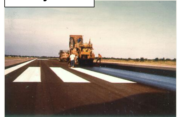
Slurry Seal
