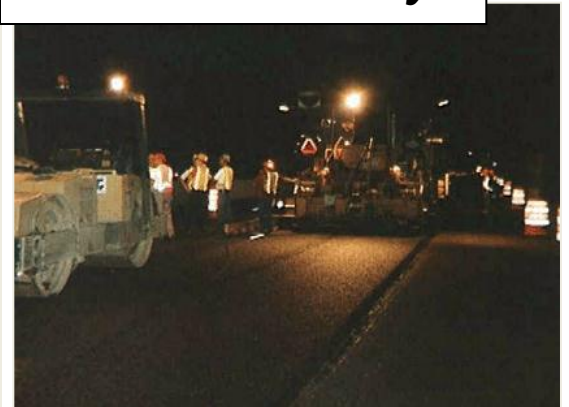
Thin HMA Overlay
