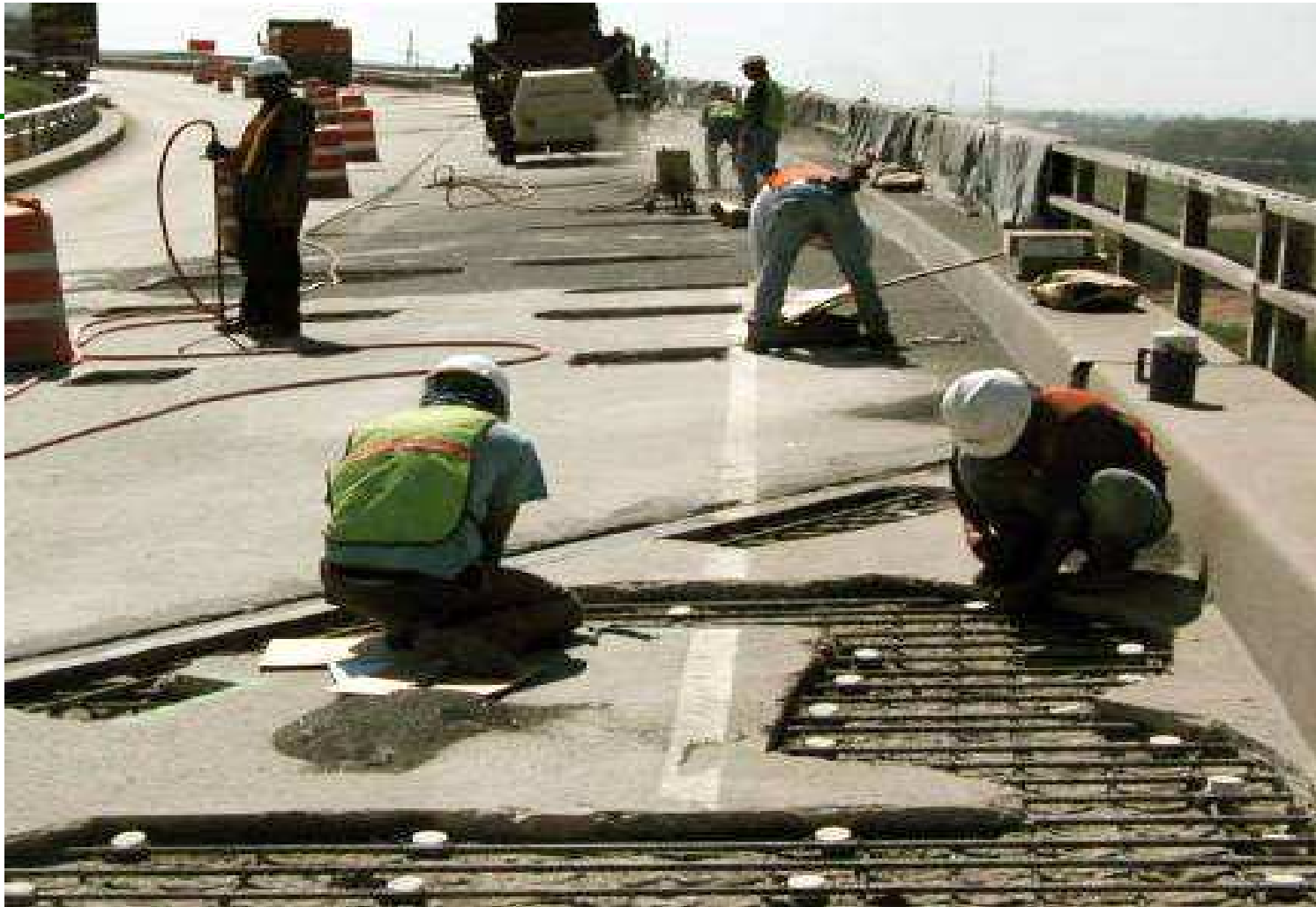
Bridge Deck - Chip and Patch Repairs. Colorado DOT – Greeley, CO
