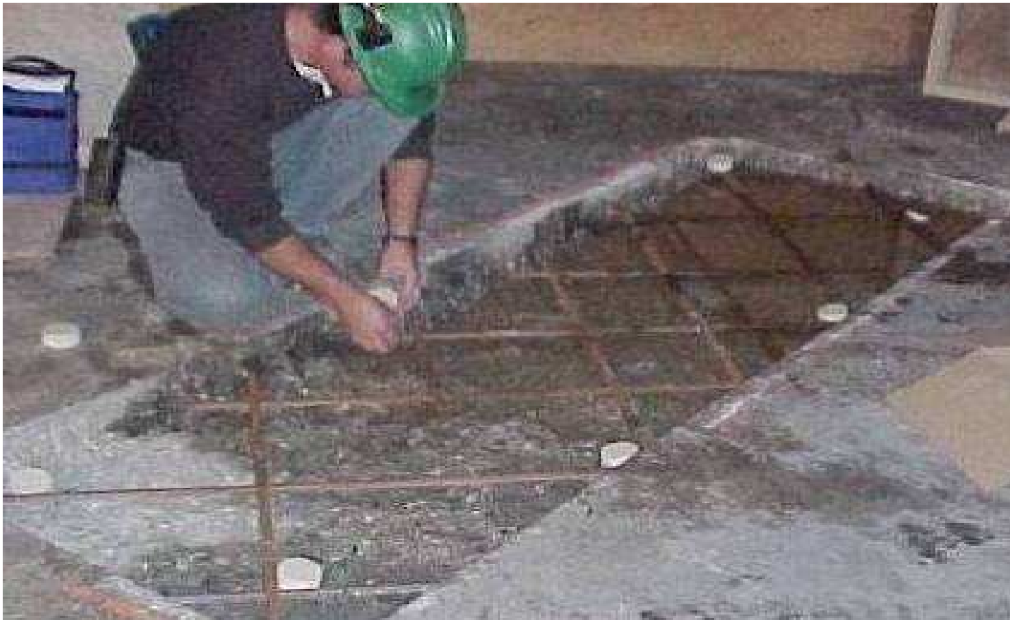
Installing anodes around the perimeter of the repair.
