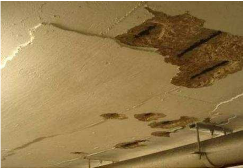
Underside of Parking Deck
