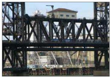
Solution – Use the moveable lower deck to inspect the upper deck floor system members at eye-level.
