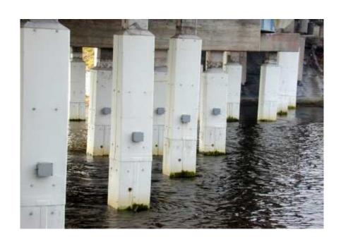
SACRIFICIAL C.P. JACKET IS PLACED AROUND THE PILE AND CONNECTED DIRECTLY TO THE REINFORCEMENT WITHOUT AN EXTERNAL POWER SUPPLY.
