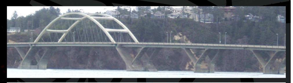
If the structure has a Y-Leg or K-frame Substructure, the Y-Leg SPAN directly above the Y-leg footing will carry that bent / span number, along with an "A" designation. The next ensuing span will carry the bent number along with a "B" designation.
