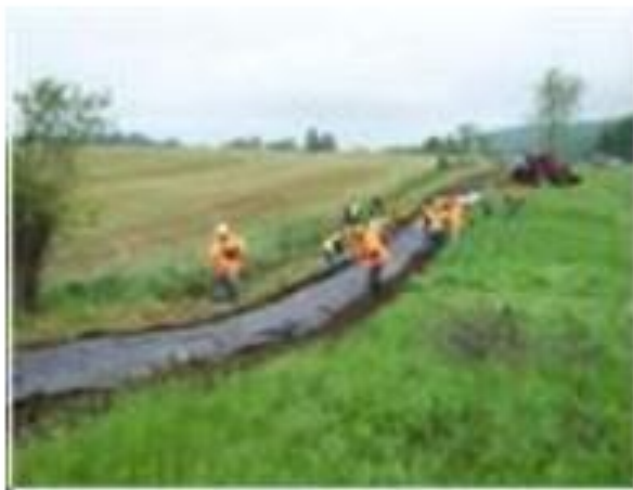
Install Living Snow fence
