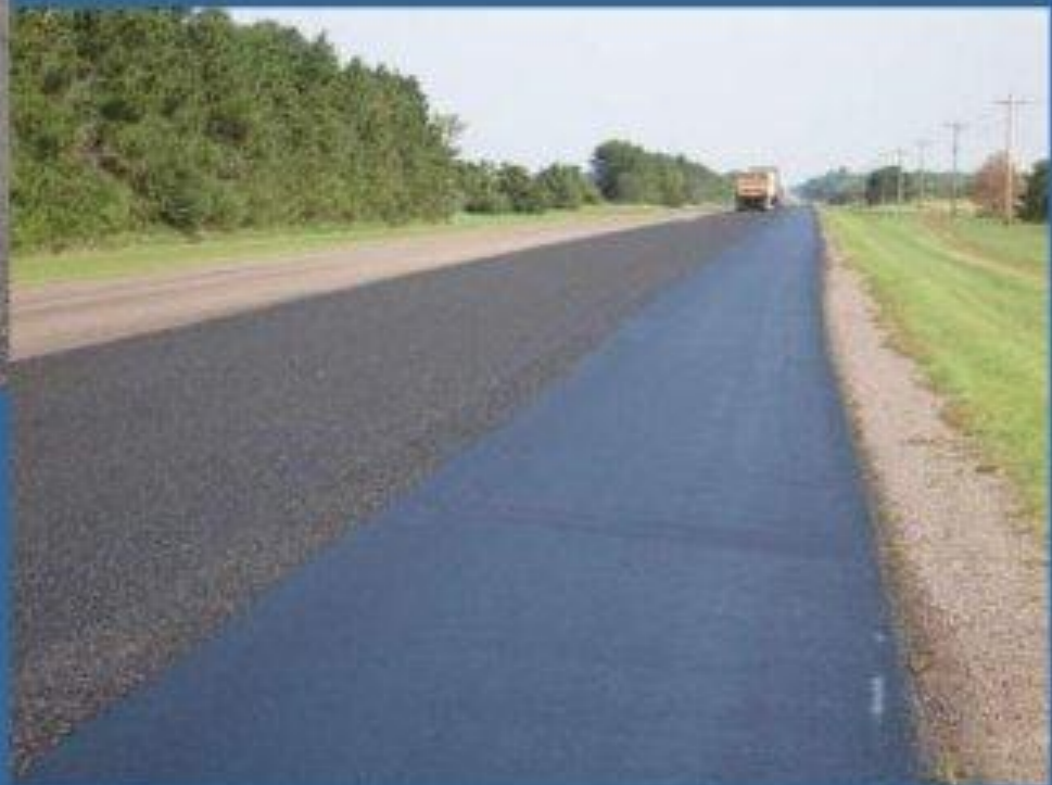
Fog Seal Application
