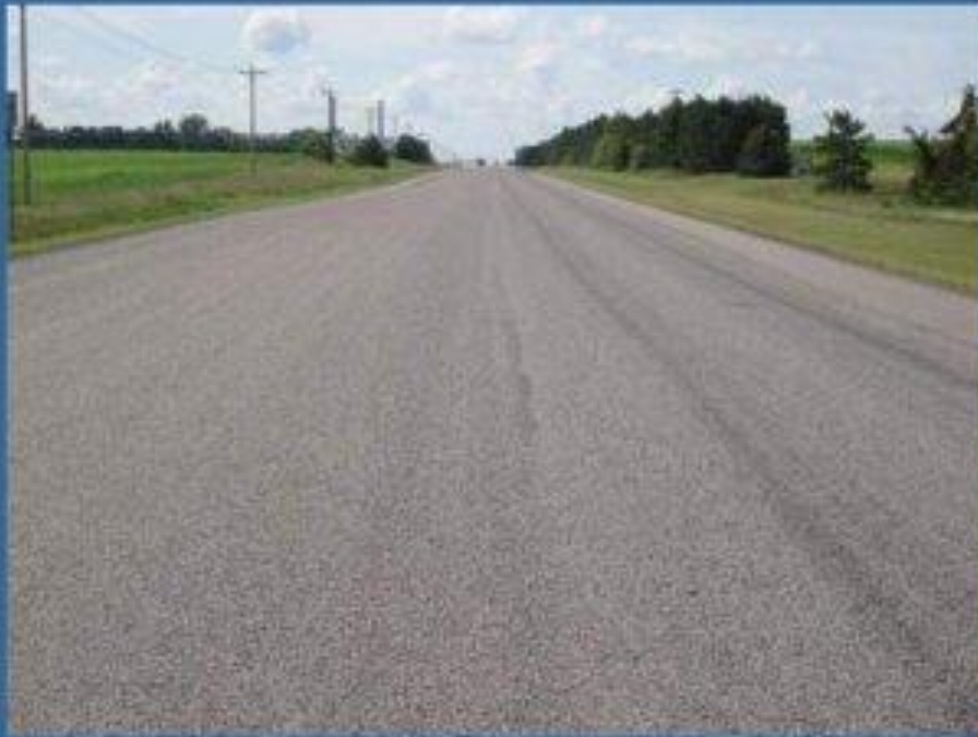
Final Seal Coat Application
