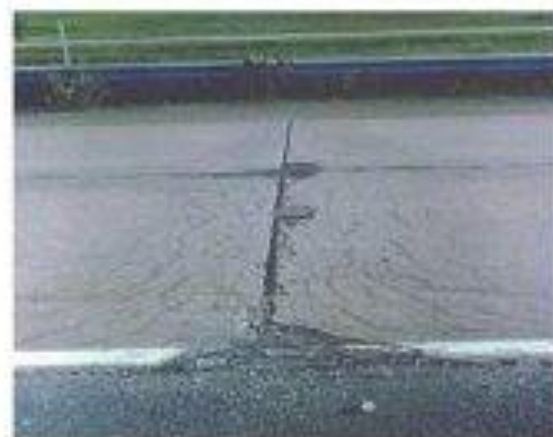
High severity "D" cracking
